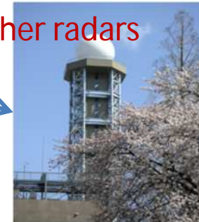
C-band Doppler Radar (5.3 GHz) JMA Standard Radar, 2006
