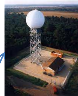
S-band Doppler Radar (2.7-3.0 GHz) WSR-88D (NEXRAD) NWS, 1988
